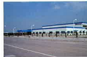
Suzhou Plant , China
