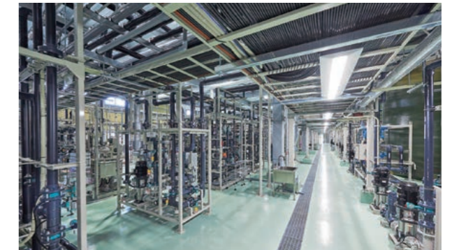
Next-generation ultrapure water system laboratory building
